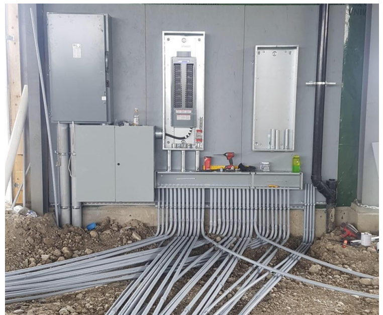
PVC 90's? Aren't you concerned about your jet line/rope cutting through them when you pull the wires? We always use rigid 90's underground.
