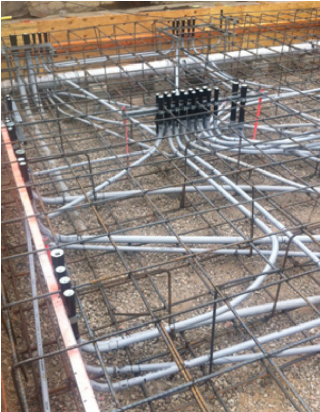
Conduit Installed in a Slab
